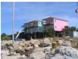
Storm water retrofit for the town of Cedar Key and new development.
